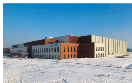
Site McPhy de Belfort (France)
