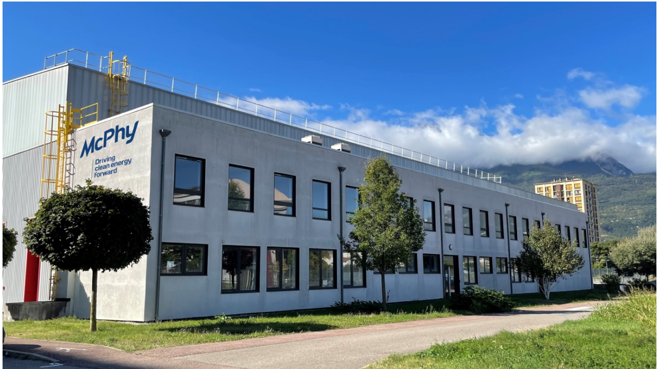
New McPhy site in Grenoble, bringing together Station activities and some head office functions
